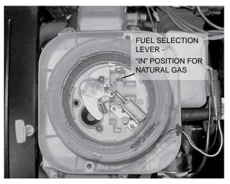
Figure 4. 12/14/16/17/20 kW, GT-990/GT-999 (Airbox Cover Removed)
